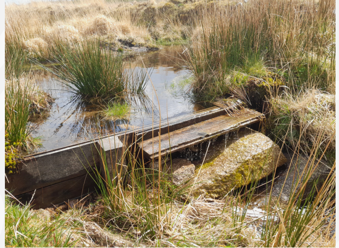
Figure 2: An example of a small leaky wooden dam. This helps to slow the flow of water, diversify wildlife habitat & improve peat health.
